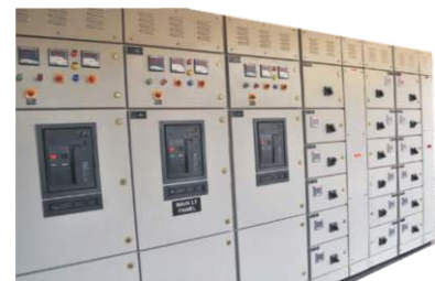
Electrical & Distribution Boards
