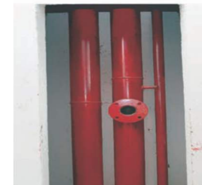
All C Class of Reputed Brands Used For Sprinkler, Hydrant & Drain Pipe ( 3 Fire Duets)
