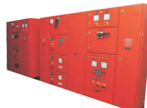
100 HP Hydrant Pump Control Panel
