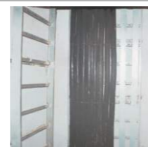
PVC Insulated & PVC Sheathed Armoured Cables 1.1 KV Grade Provide Upto Each Floors
