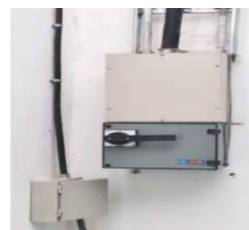
L.T Main switch Per Unit
