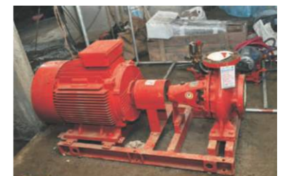
Hydrant And Sprinkler Pump Of Kirlosker Make (92HP)
